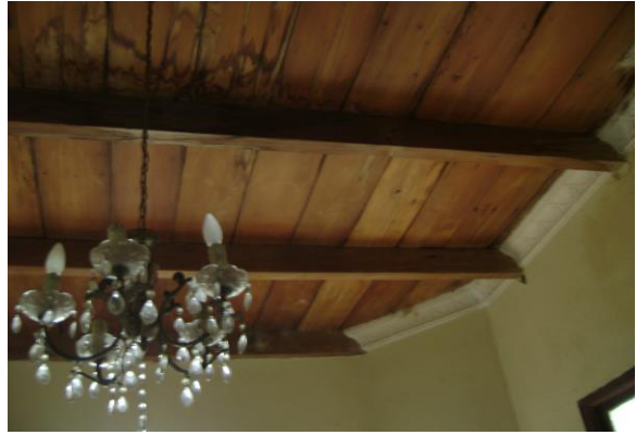
Fig 6: yellowwood ceiling in dining-room
