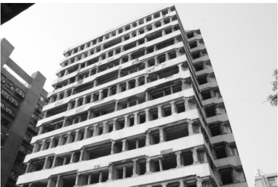
Skipper Tower, 22, Barakhambha Road
